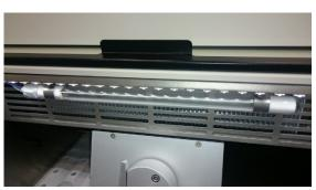
Once the plug is connected to the UV- Lamp, the final step can be done now and the UV-Lamp unit can clip into the retaining clips.
